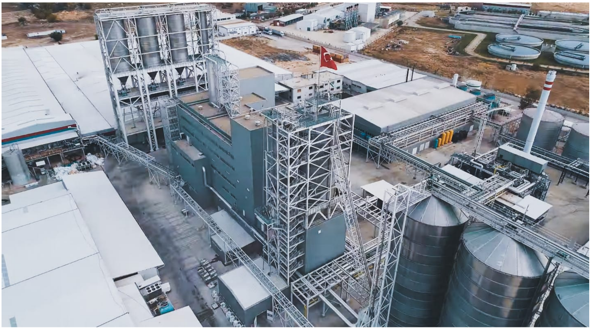
PET production line built by thyssenkrupp in 2013
