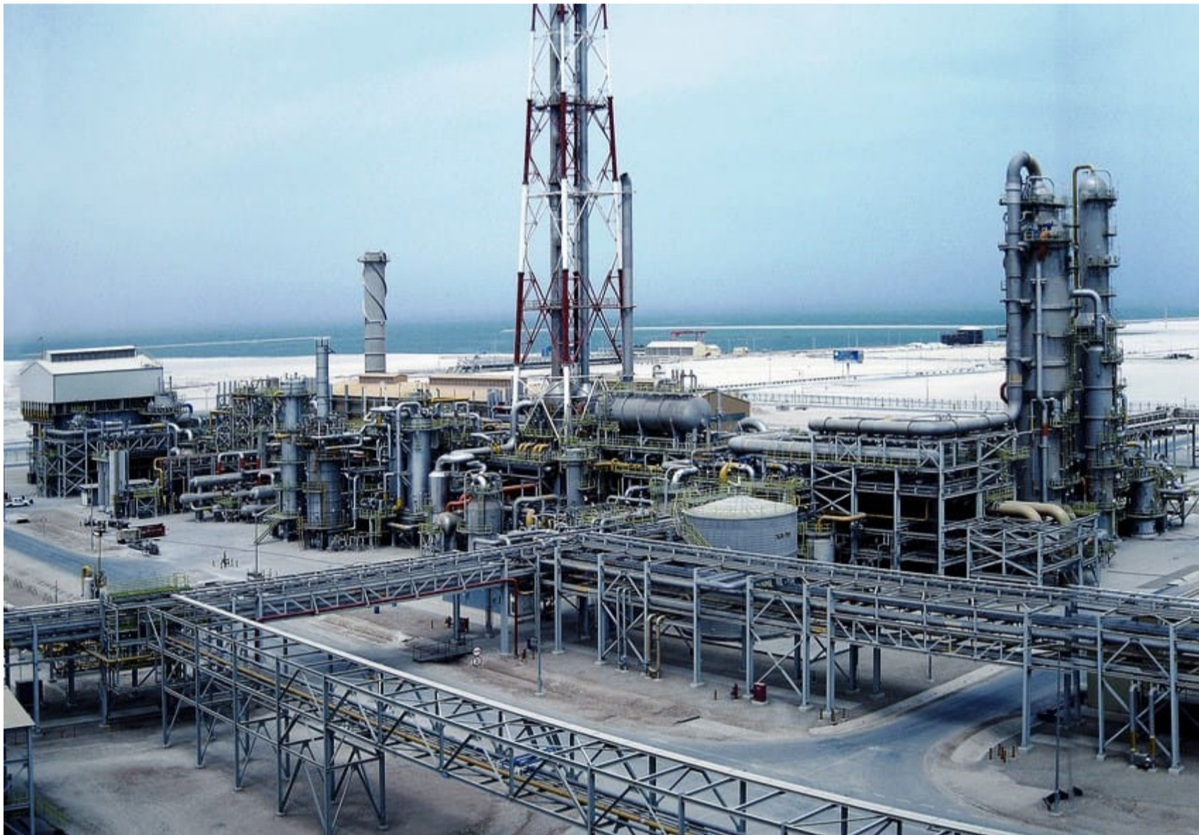
Ammonia plant Ma'aden 1
