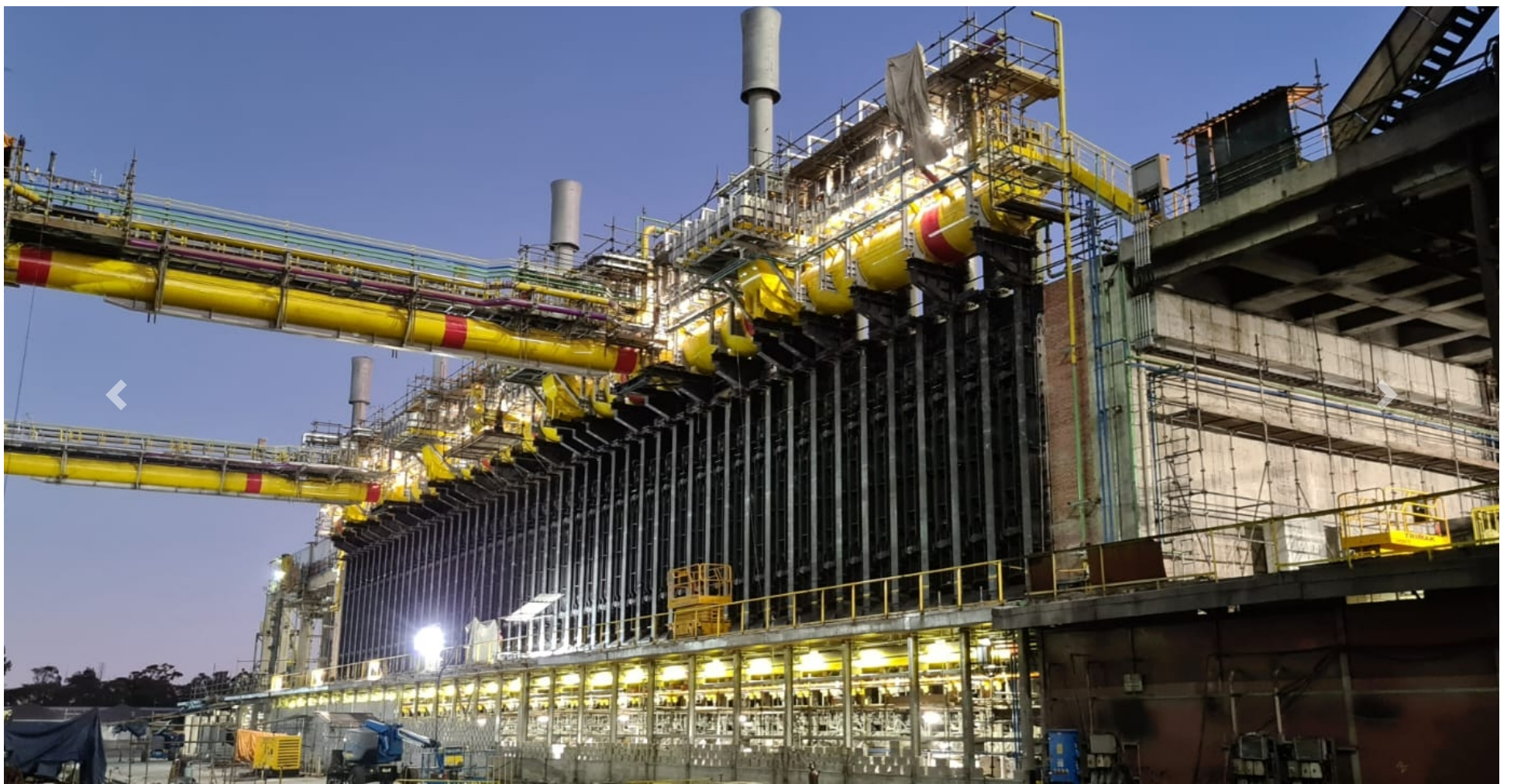
New coke oven battery
