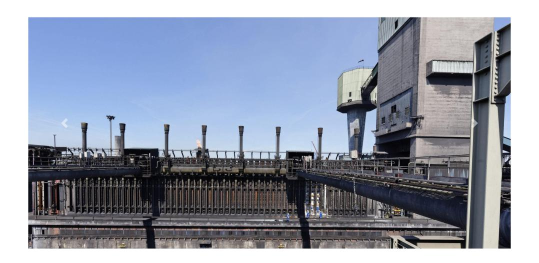
The bottom line: The flue-end repairs on two coke batteries at the ArcelorMittal Coking Plant in Ghent were so extensive they took over five years to complete. Besides demolishing and reconstructing the ovens' 102 refractory walls, buckstays, doorframes and doors were replaced or refurbished. The work was carried out to the customer's complete satisfaction by thyssenkrupp Uhde Engineering Services and its subcontractors – with no major accidents at any time.
